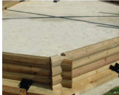
Lay out the base structure and start to build the wooden sections which fit together perfectly
